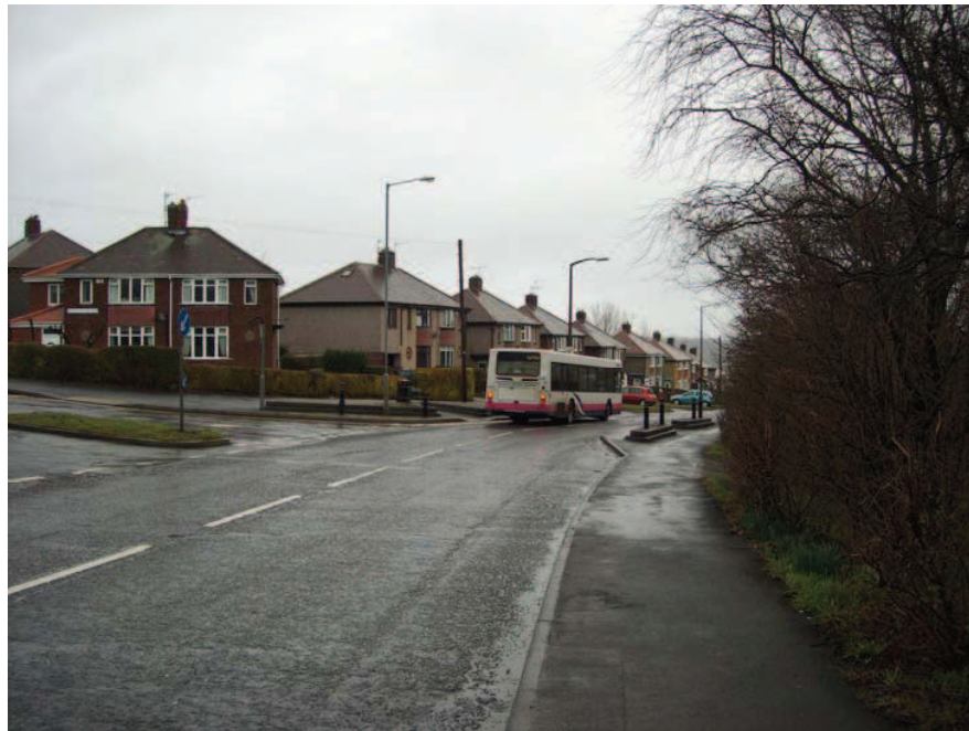
The bend restricts road user intervisibility
