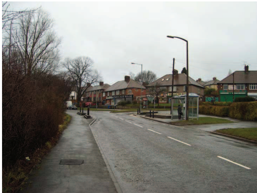
The existing build out – the inbound bus stop can also be seen
